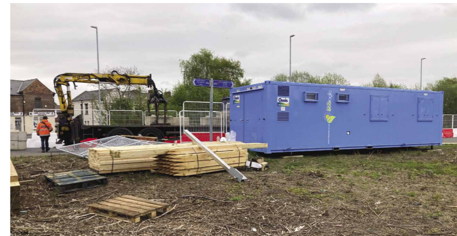
Above: A site office and fencing materials have also been delivered.
