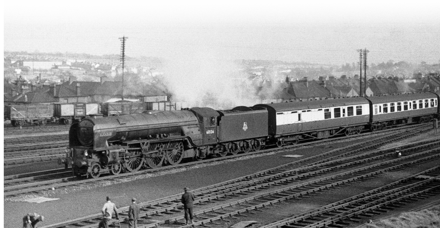
No. 60136 Alcazar on a down train approaching New Barnet Station in 1957.
