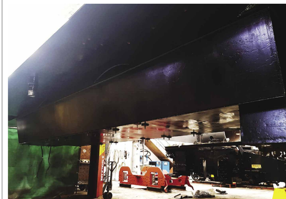
The underside of the tender has been cleaned and painted by Ben Poole. After cleaning the bare metal areas and painting in primer, and after a few coats of undercoat, a coat of black gloss is applied - the bogie frame in red primer can be seen in the background.
