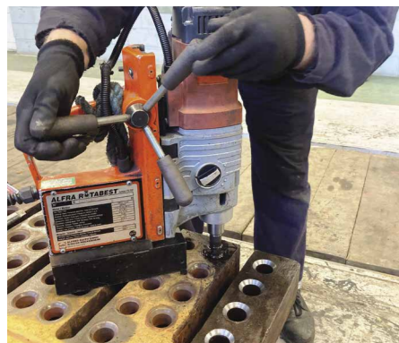
Above: Re-cutting the seats on the superheater header.
